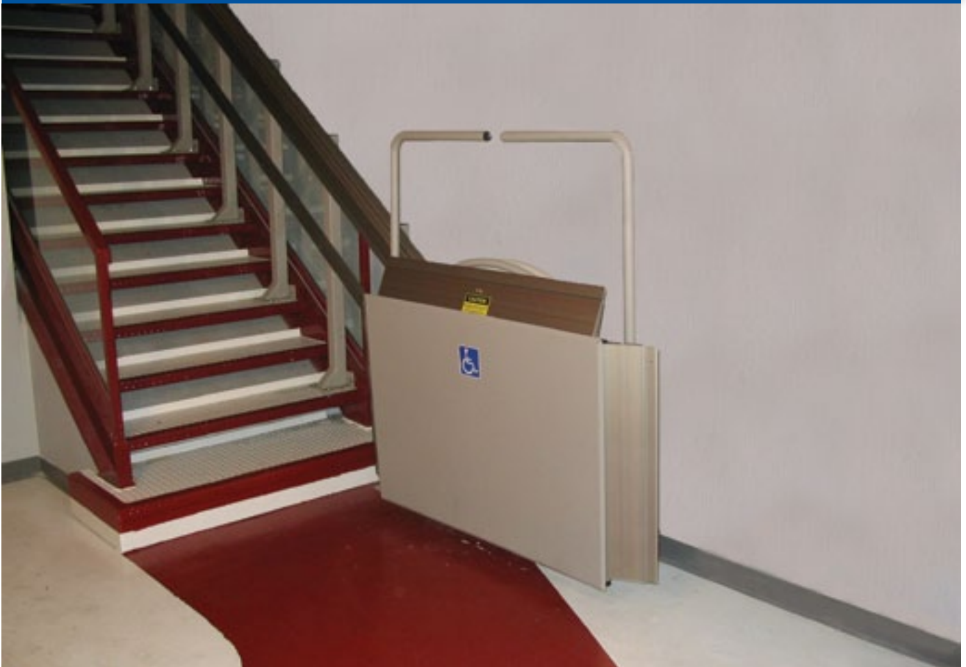
Inclined platform lift for straight stairways
