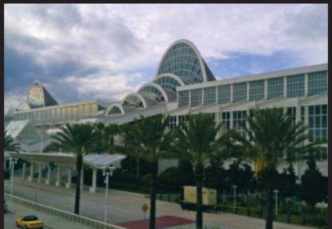
Orange County Convention Center - Orlando
