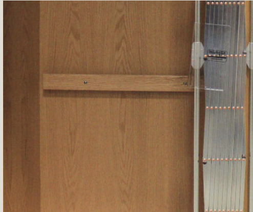
Standard wood handrail matches wall finish.
