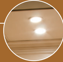
LED ceiling lights
